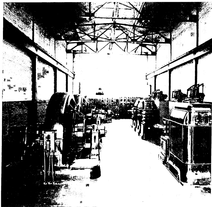
FIG. 6. A converter substation containing synchronous converters. Note that no separate motor is required to drive such a converter. The General Electric Co.
