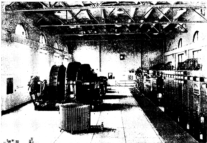
FIG. 5. A converter substation containing motor-generator converters for the purpose of converting the alternating-current power to direct-current power to be used by locomotives in the Detroit Tunnel.
